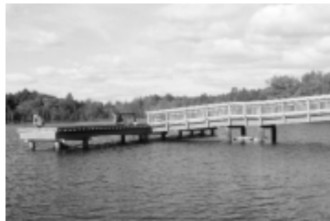
Accessible fishing pier with ramp at Carboncle Pond in Rhode Island
