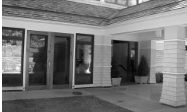
Doors with glass side panels allow for natural light and make it easy to see someone at the door.
